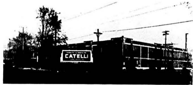
Exterior view of the Catelli Food Products plant in Montreal, Canada's largest and most modern macaroni factory.
